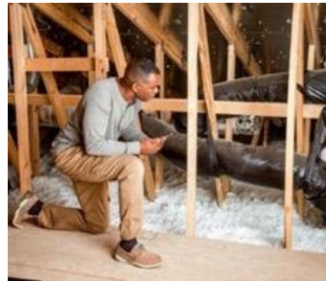
Attic & Wall Insulation
